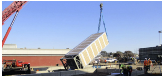
Richmond HS - Installing Science Building Elevator
