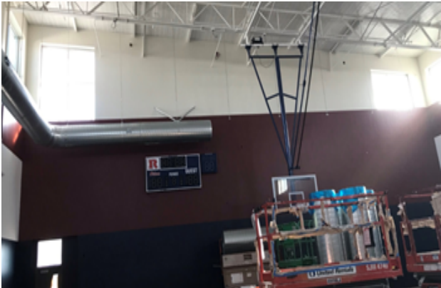
Interior of new gym
