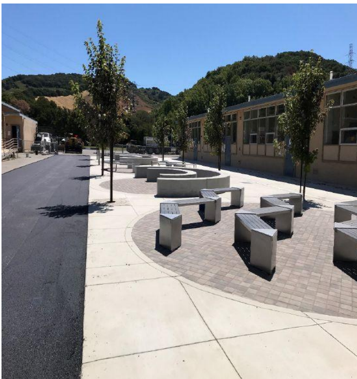
Olinda Elementary School - repair tripping hazard due to tree roots lifting concrete
