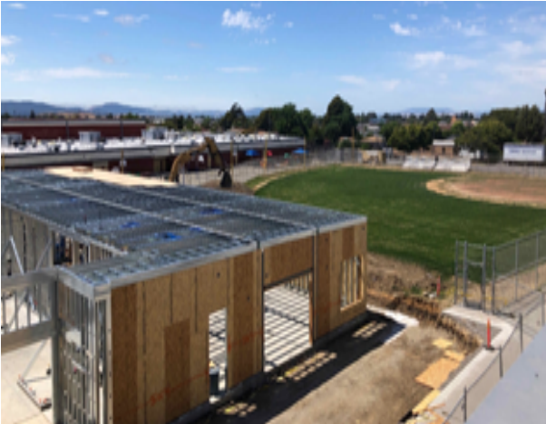
Aerial View of Framing of New Gym
