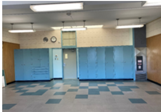
Painting Ceiling, Walls & Trim Classroom in Building 500
