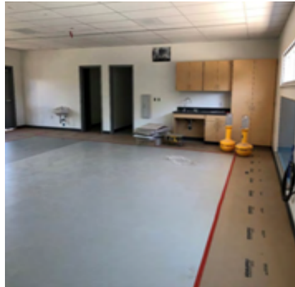
Pre Kindergarten Flooring
