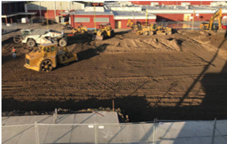
Richmond HS - Soil Compaction for Gym Pad
