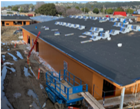
Roofing – Admin, Kinder North & South
