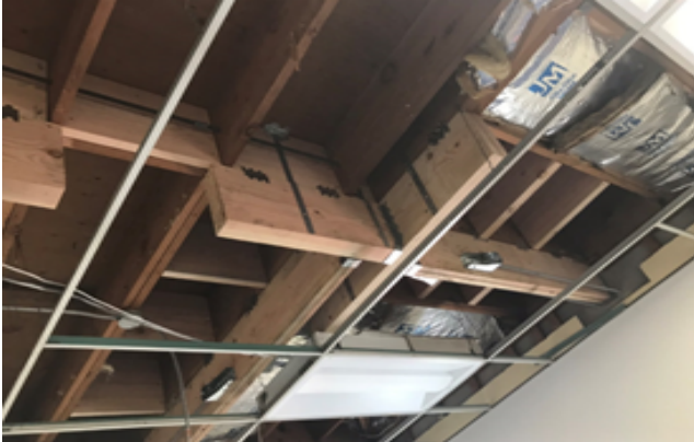
Seismic Blocking – Science Building
