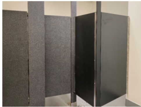
New ADA compliant bathrooms (Critical Need Phase 2)
