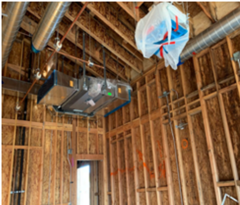
Administration Bldg. - HVAC Ducts
