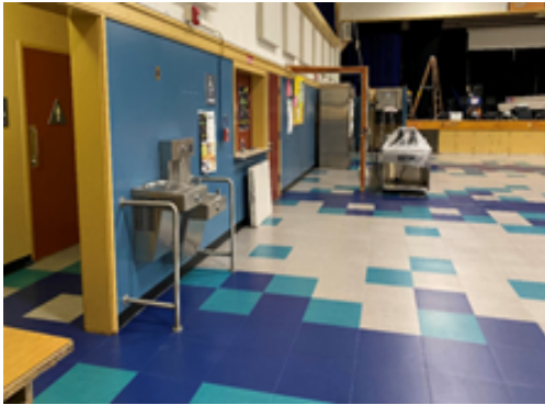
Multipurpose Room Tile (Critical Need Phase 2)
