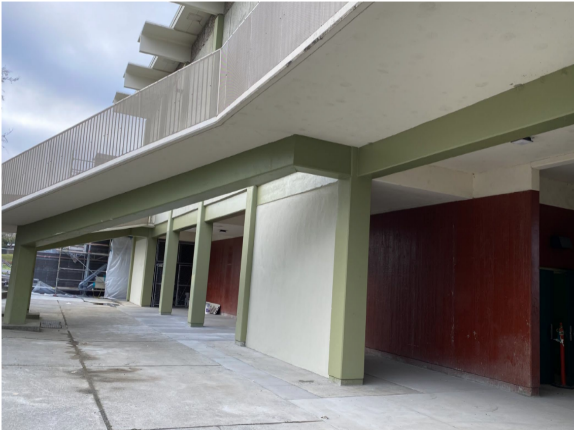
Juan Crespi Middle School - Gym Seismic Retrofit - Shear Wall Outside Gym 11
