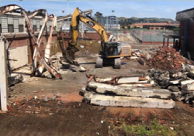
Old Gym Demolition
